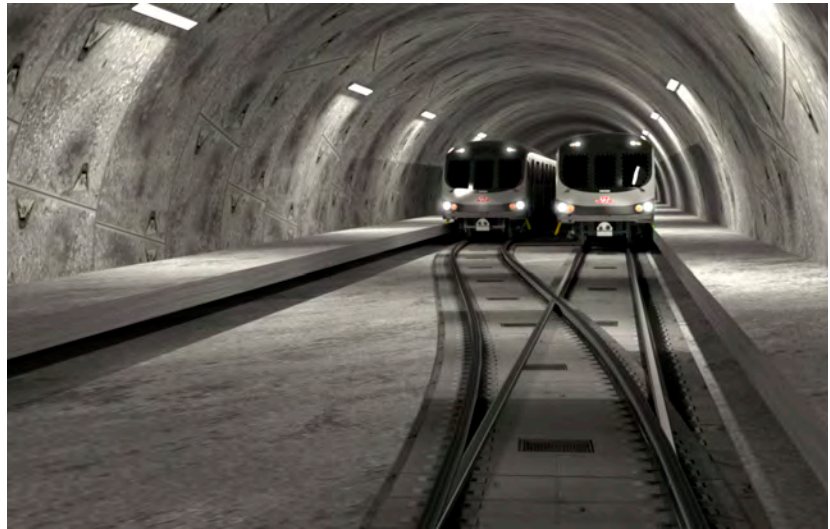
Scarborough Subway Extension, Toronto, Ontario: Large diameter transit tunnel with double track configuration - design implementation in progress on the Scarborough Subway Extension.
