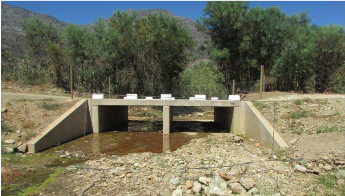
6m Causeway (Loop River Structure – C960.1)
