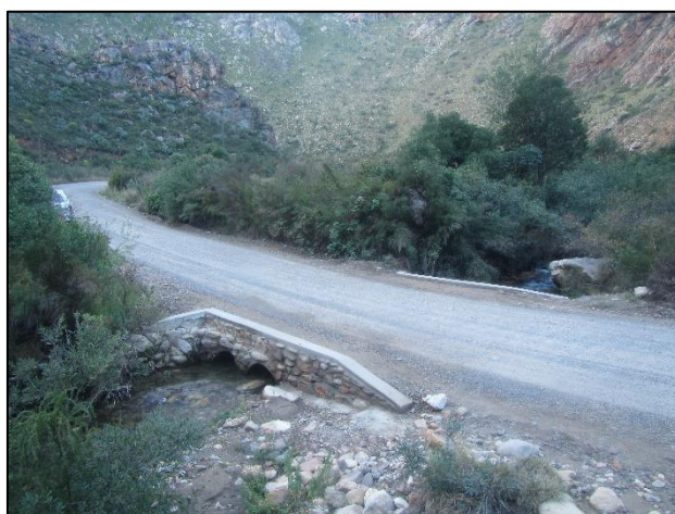
Current river crossing at km 54.1.
