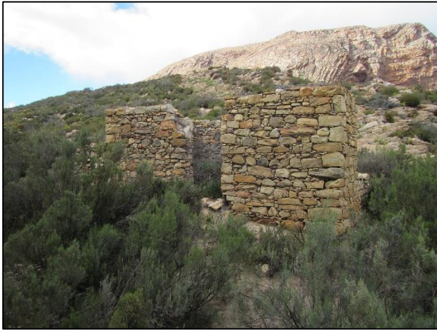
Figure 14: Ruined structure at waypoint 255.
