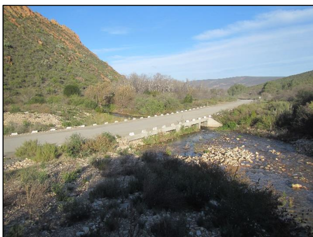
Current river crossing at km 57.1.
