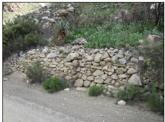
Drystone retaining wall with mountain slope above and road below (waypoint 250).
