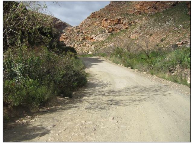
Current river crossing at km 47.2.
