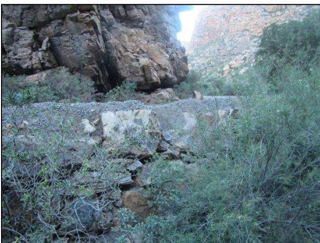
Drystone retaining wall with road above and river below (waypoint 217).
