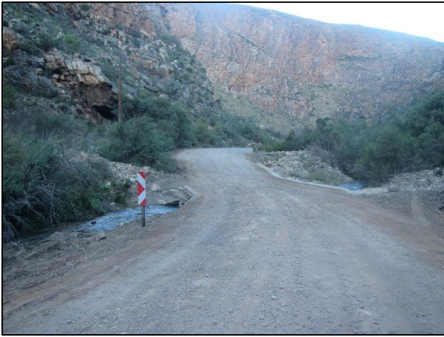
Current river crossing at km 53.4.
