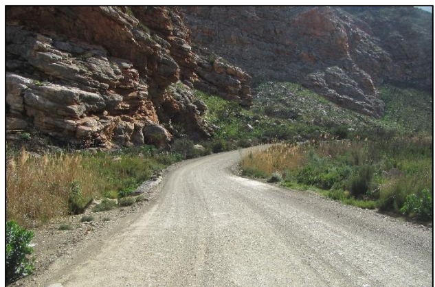
Figure 7: Current river crossing at km 44.3.
