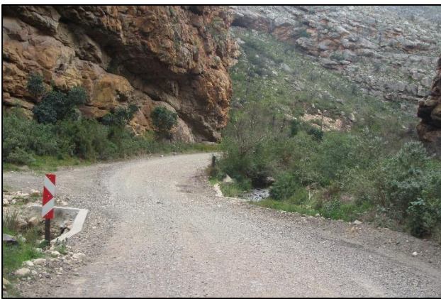
Current river crossing at km 50.8.
