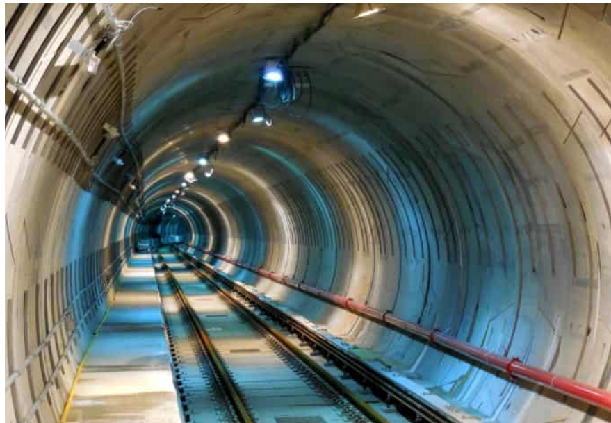
Spadina Subway Extension, Toronto, Ontario, Canada
