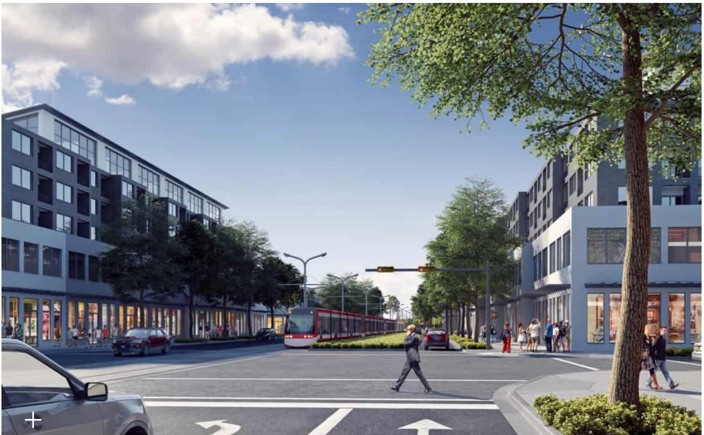
Green Line LRT, Calgary, Alberta, Canada
