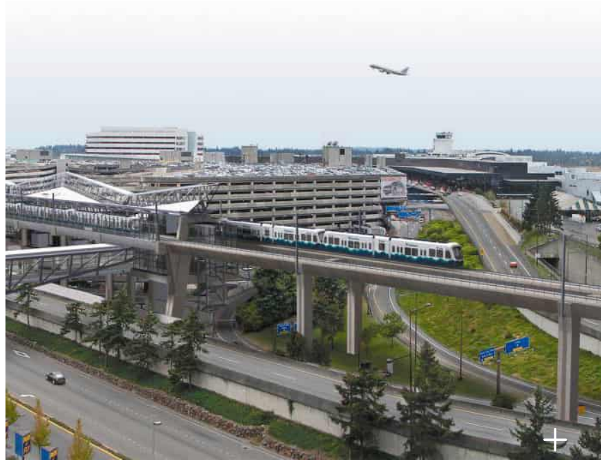
Sound Transit Central Link, connecting downtown Seattle with the city's airport
