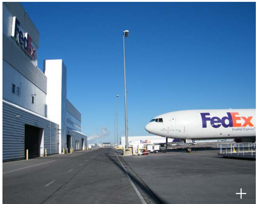
FedEx Canada facility
