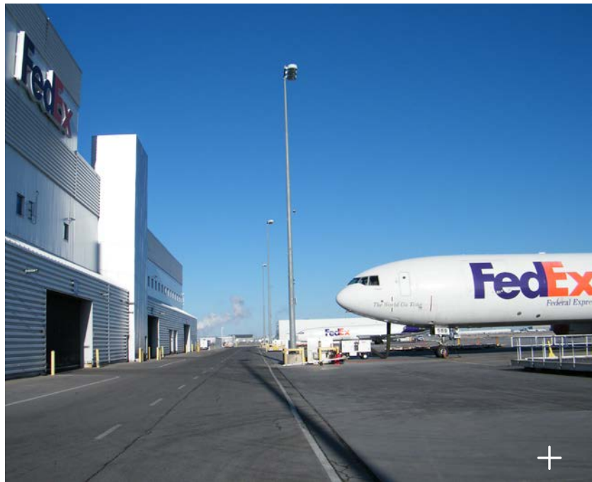
FedEx Canada facility
