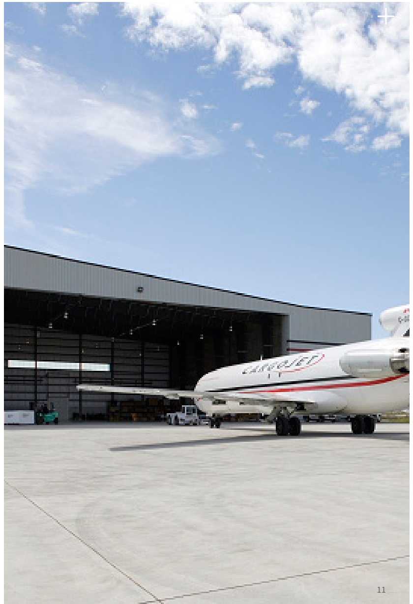
Cargojet maintenance hangar, Hamilton, Ontario
