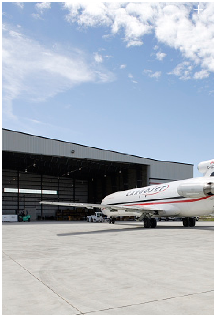
Cargojet maintenance hangar, Hamilton, Ontario
