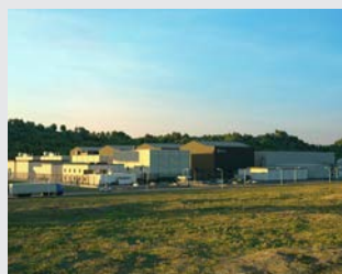
Xe-100 Technology Development Program Engineering Support Services
