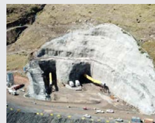
Lesotho Highlands Water Project Polihali Dam Diversion Tunnels
