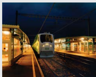
GO Expansion - On-Corridor Works
