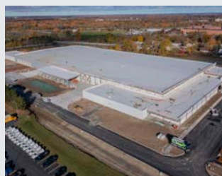
Li-Cycle Hub Warehouse
